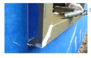
ThermalBuck features an integrated sill pan with a slope of 1/16" on all 8' lengths.
