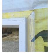
Release head flap of WRB and press into sealant. Smooth to remove all wrinkles.
