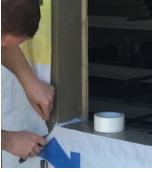
Angle all four corners to pull head and sill flap back .
