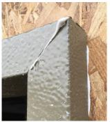
Repeat for each jamb, and head piece. Ensure all 4 corners align, and adjust as needed. 100% oozeout is needed at all transitions for proper water and air sealing.
