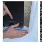
Flash across both ends of the horizontal flashing across the sill, to cover the end of the WRB.
