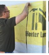
**CUT WRB** Cut all 4 sides of WRB flush to Rough Opening.
