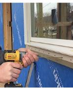
**NOTE:** Fasteners must penetrate min 1-1/4" into structure.
